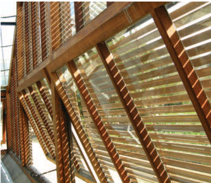
Cedar shading installed to Mountains display in Alpine House, thanks to a grant from the Hendry Bequest of the Alpine Garden Society
