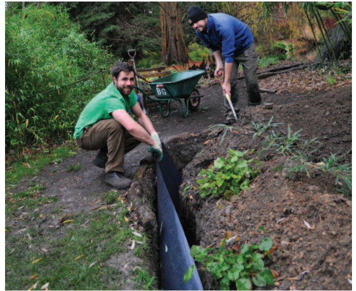
DIGGING IN THE NEW RHIZOME BARRIER ALONG THE STREAM
