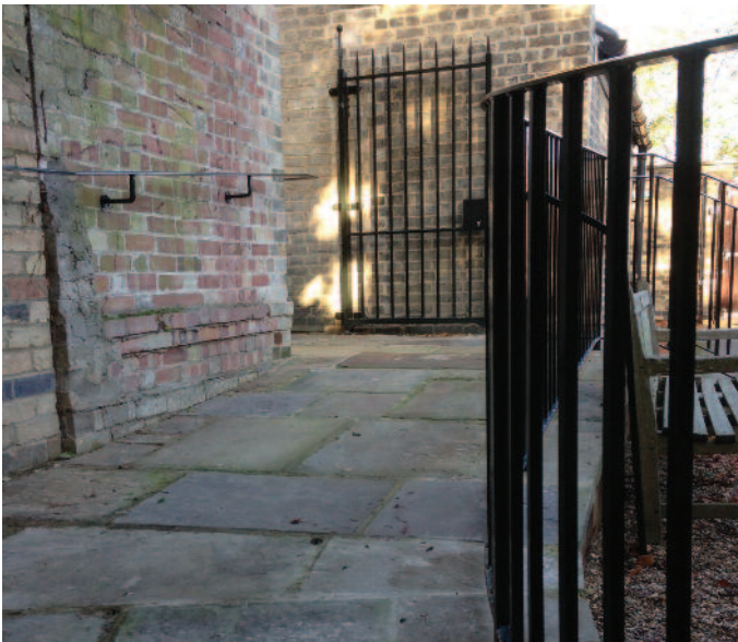
The new ramp en route to Brookside
