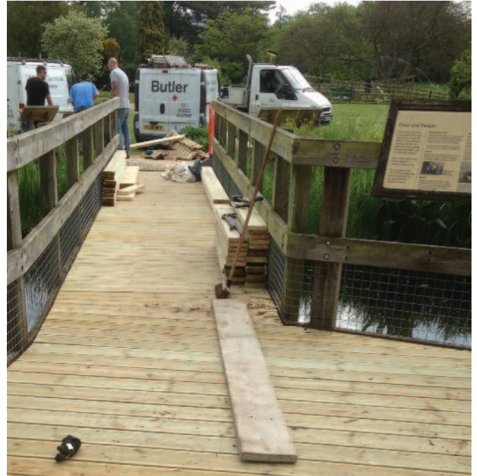
FENLAND BRIDGE NEW DECKING
