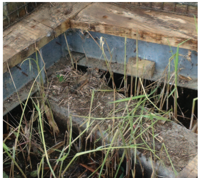
FENLAND BRIDGE TIMBER REMOVED
