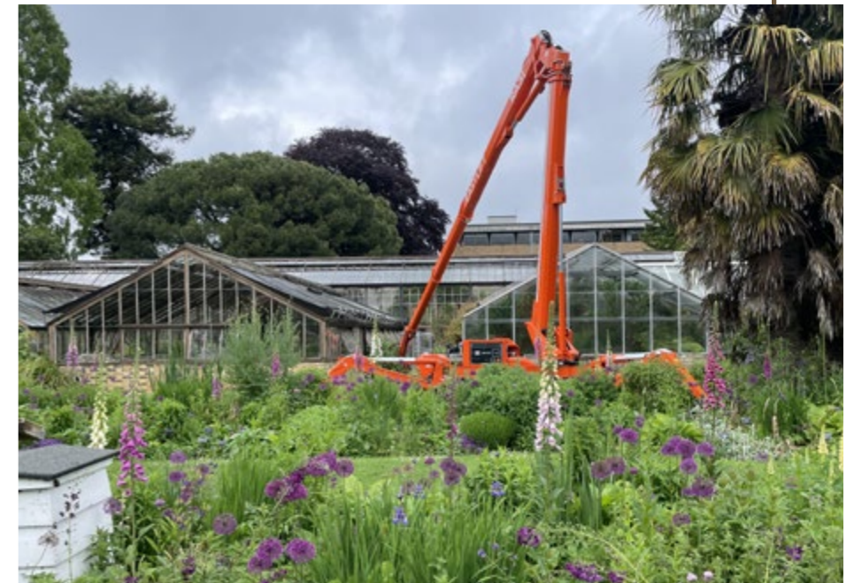
Crane work on the Glasshouse Range
