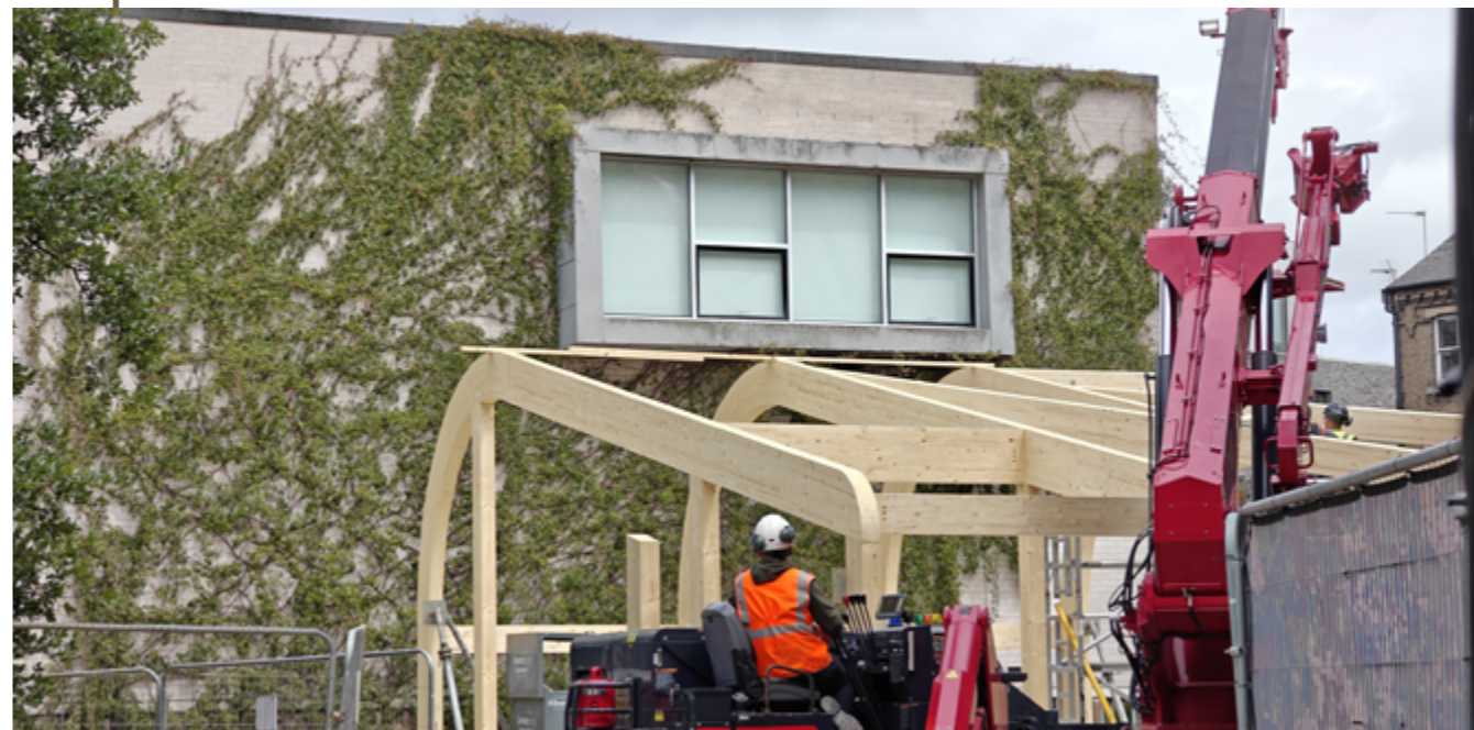
Station Road ticket office progress
